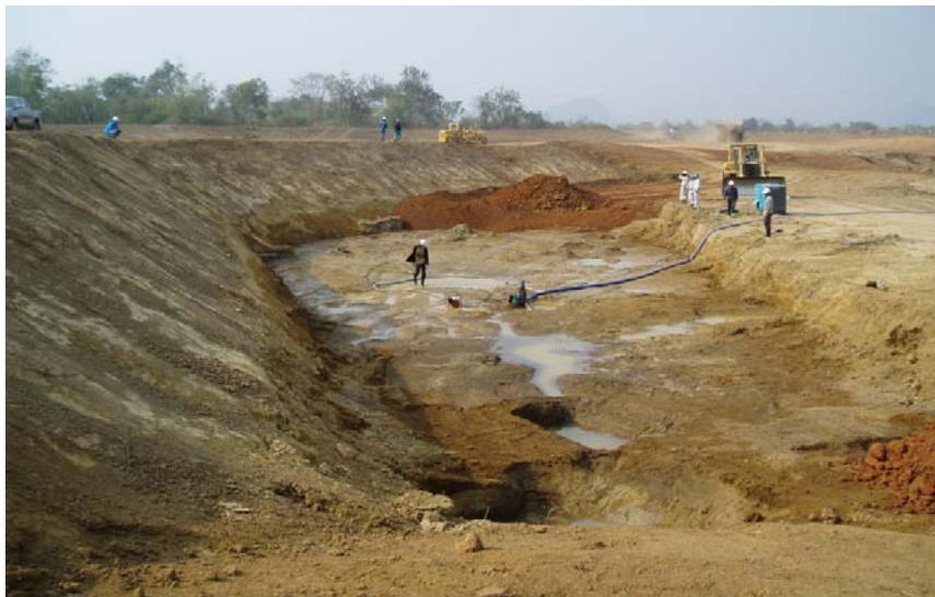
Typical downstream channel construction
