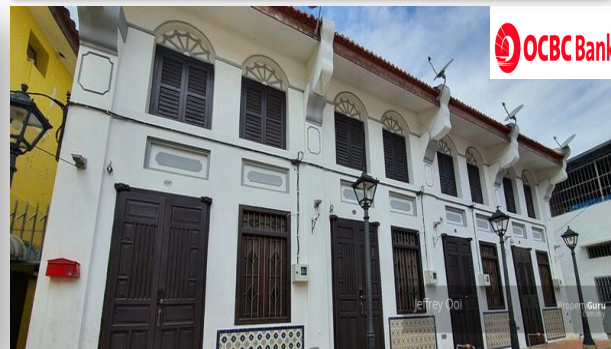
Refurbishment of Shop House, Lebuh Pantai, Penang for OCBC Bank (M) Berhad.
