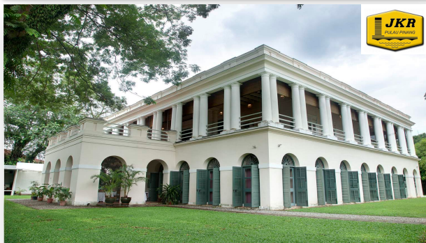
Refurbishment of Suffolk House Penang (Phase 2) for JKR Pulau Pinang.
